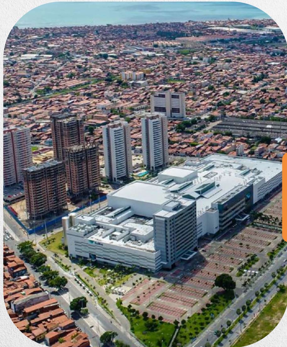
BOULEVARD SHOPPING RESIDENCE - CE
